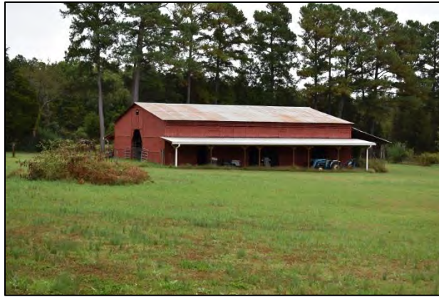
Figure 29: Side (eastern) elevation of barn.
