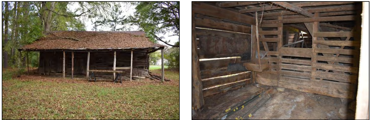
Figure 11: Left, view of front (southern) elevation; right, interior view looking to north.
