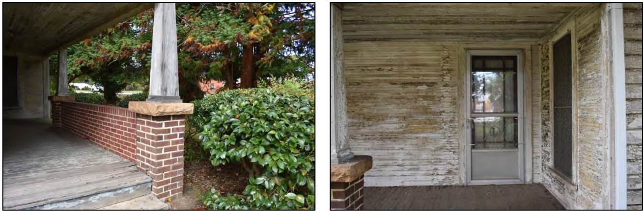
Figure 6: Details of the front porch.
